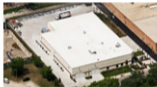
Meridian Design Build completed an approximately 37,942-square-foot warehouse/distribution facility for Gypsum Supply Co. in Chicago.
