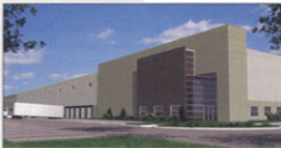
Meridian Design Build will construct the third building in Bluff Point Business Park in Romeoville, Ill.
