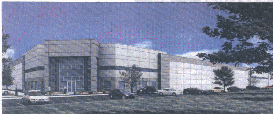
TCB Development and Tobin Development are building this 574,249-sq.-ft. distribution center in Midpoint USA in Portage, Ind. Leasing activity should pick up in Northwest Indiana once 1.2 million sq. ft. of industrial comes online there this year.
