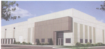
DP Partners broke ground on this building, its third speculative building at LogistiCenter at Sauk Village.
