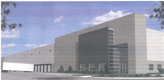
Land and Lakes Development Co. broke ground in early August on this 506,777-sq-ft industrial building in the Bluff Point Business Park in Romeoville. This nearly 1 million-sq-ft freezer cooler building is under construction for Central Grocers in Joliet.
