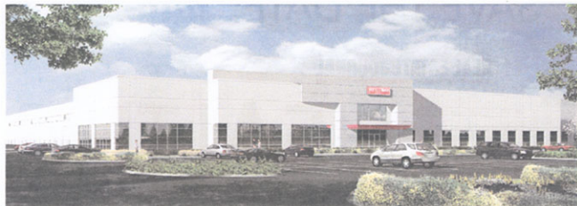
Auto Truck Group and Abbott Land and Investment Corp. selected Meridian Design Build to construct its corporate office/showroom/manufacturing facility in Bartlett.
