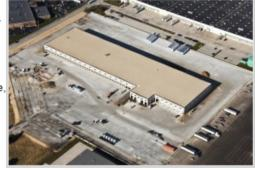
crushing/recycling of more than 14,000 tons of asphalt and concrete. Existing light duty pavement was left in place to the extent possible and topped with Roller Compacted Concrete to accommodate the new use. The completed facility includes a full-service truck maintenance shop, a truck wash, 500 leased trailer positions and a diesel fueling island designed to allow the growing company to provide comprehensive services to its third party clients.
