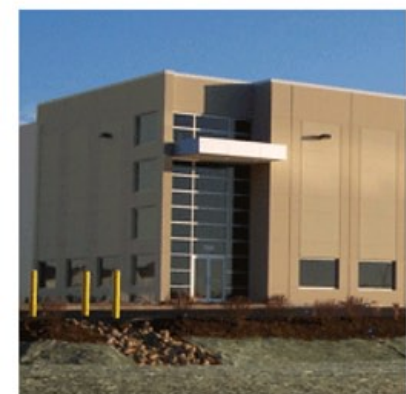
Danfoss' new facility
