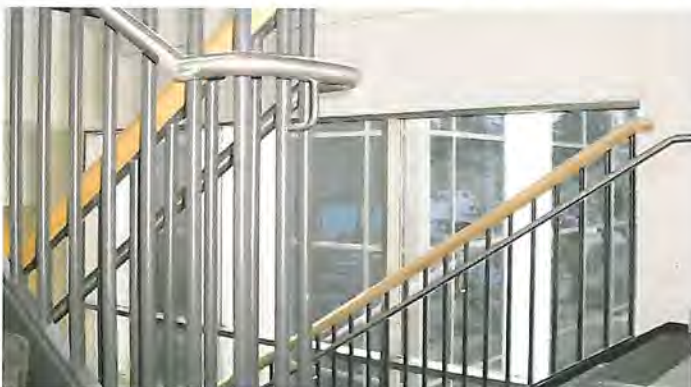
Photo courtesy of Meridian Design Build LLC
