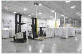
upgraded throughout the climate controlled facility to incorporate energy efficient T-5 lighting with motion sensor controls.
