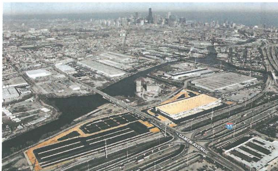
Aerial view of the new 219,858 SF automated package sortation and distribution center Meridian recently completed for developer Scannell Properties at I-55 and South Damen Avenue.
