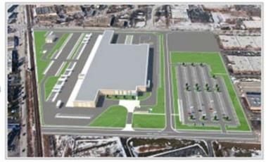
The project will include demolition of an existing 756,000square-foot building and adjacent parking lots. More than 50,000 tons of concrete will be crushed onsite and recycled to reduce environmental impacts and minimize overall project costs.
