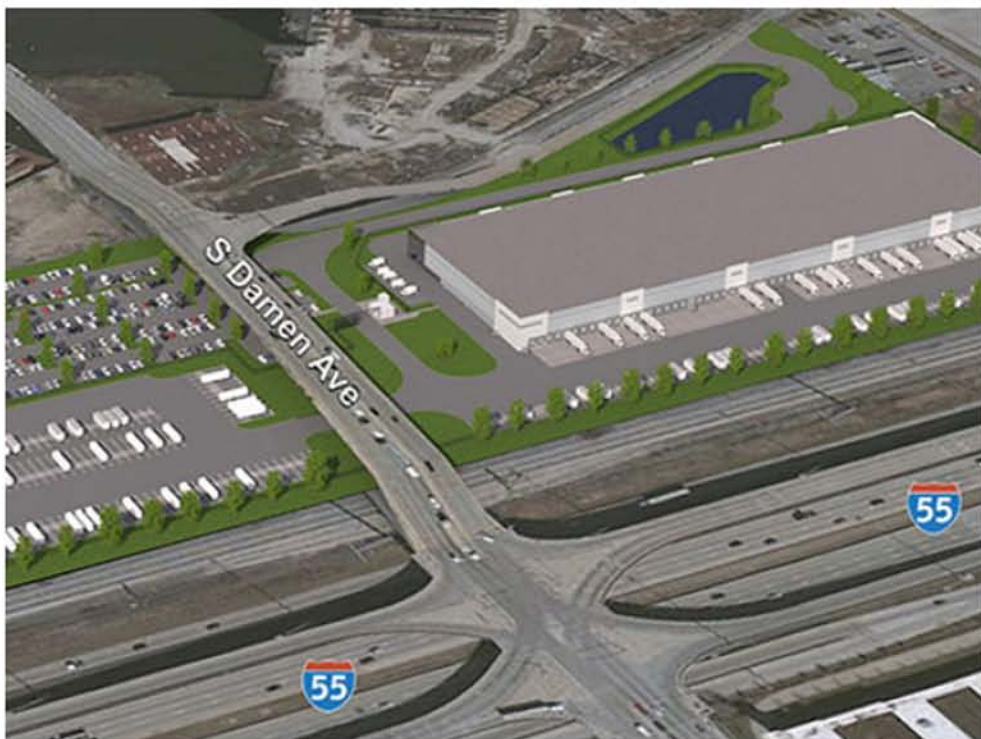
Aerial view of the site in Chicago for the new 219,858-square-foot automated package sorting and distribution center
